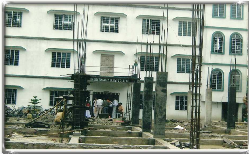
Re construction of College Building (Main)
